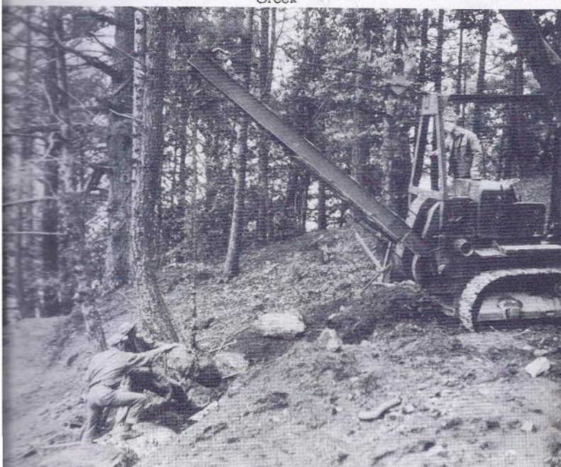
Placing Rock in Retaining Wall
