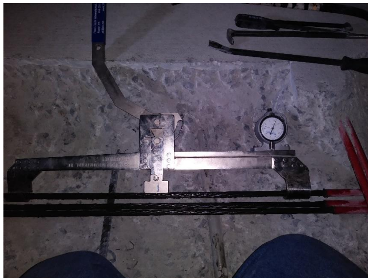
Fig 3: Tension Meter Installed on Tendon 91C
