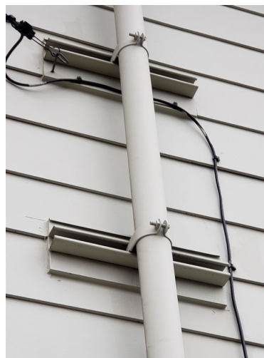
Figure 3.7.1.1f. Kindorf Bracket Attachment
