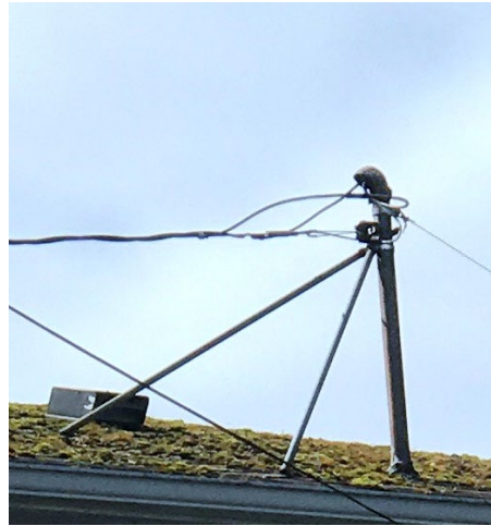
Figure 3.7.1.1f. Kindorf Bracket Attachment
