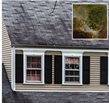
Gloeocapsa magma is blue-green in color, but surrounds itself with a dark brownish-black shell to protect against the sun's rays. The dark shell causes the telltale streaking on the roof.
