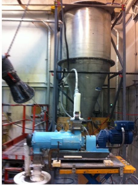
Figure 13. Air-assist hopper, double-diaphragm pump, transfer chute, and pin mixer.
