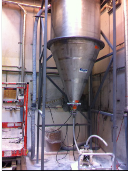
Figure 12. Air-assist hopper and double-diaphragm pump for handling fumed silica.
