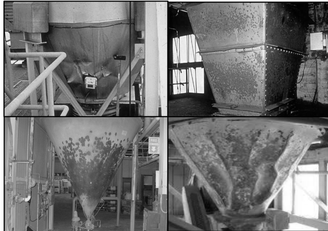
Figure 1.1. Examples of “bin rash”.
