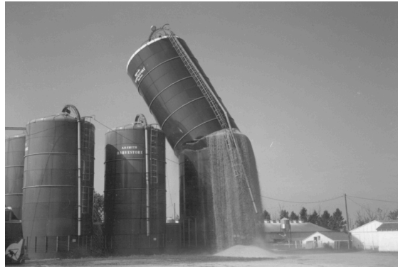
Figure 3.10. Example of silo failure.
