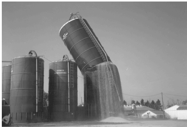
Figure 3.11. Example of silo failure.
