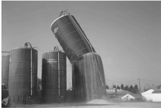
Figure 3.10. Example of silo failure.
