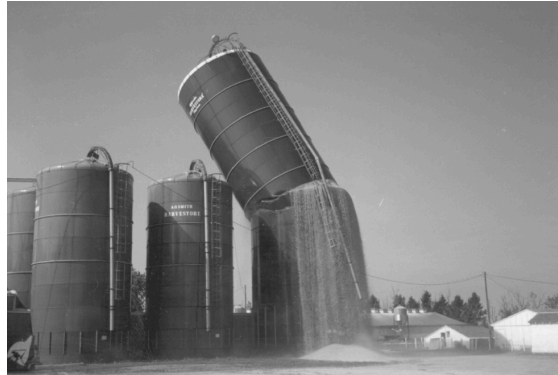
Figure 3.10. Example of silo failure.
