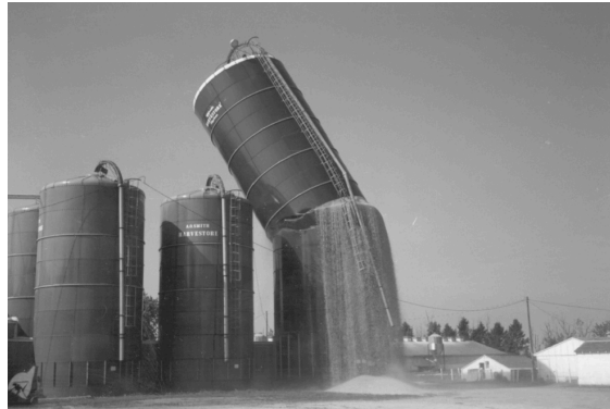
Figure 3.10. Example of silo failure.
