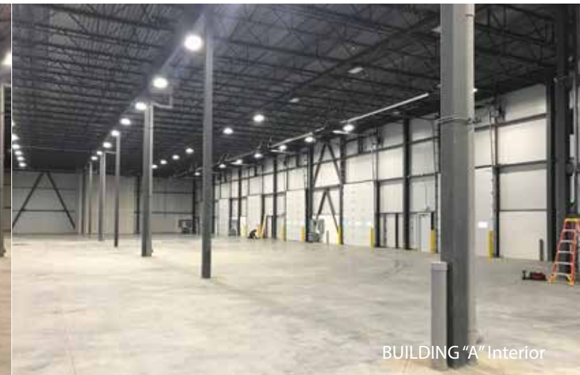
BUILDING "A" Interior
