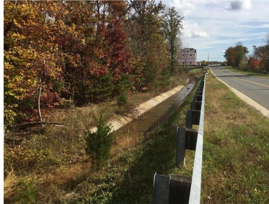
*Ditch and guardrail next to road may impact placement of sidewalk on the east side of the project corridor*
