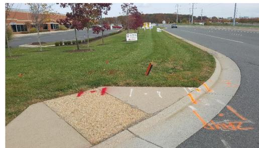
*Curb ramp upgrades are required, and underground utilities run along the length of the project corridor*
