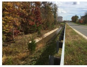
Ditch and guardrail next to road may impact placement of sidewalk on the east side of the project corridor
