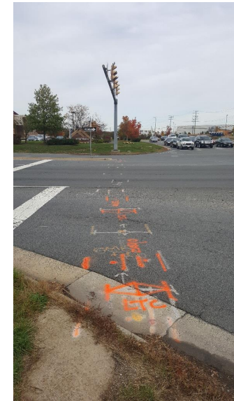
Utility lines cross the west side of the intersection
