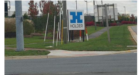
Some existing curb ramps will require upgrades, while others will remain
