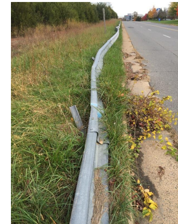
Guardrail in location of proposed path
