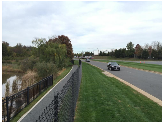
Fencing along private property may limit available right-of-way for path in some locations
