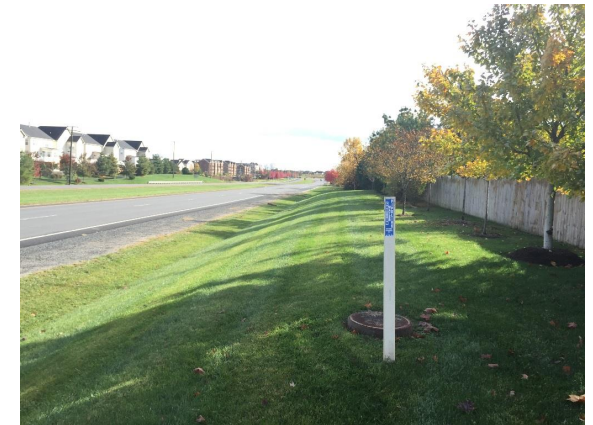
Several underground utilities lie in the right-of-way of the Alternate Project
