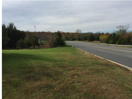
Existing wetlands and culvert may impact placement of proposed sidewalk
