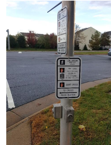
Existing obsolete pedestrian push-buttons
