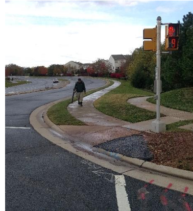
Existing curb ramps at the intersection should be upgraded to meet ADA standards
