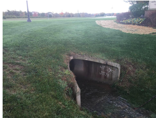
The Proposed Project will navigate around a steep slope and culvert
