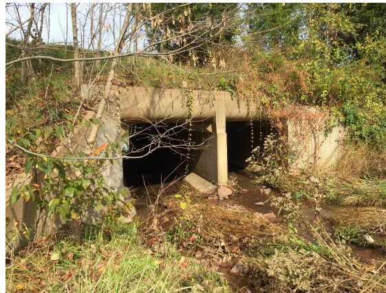
Existing box culvert on south side of Prentice Drive
