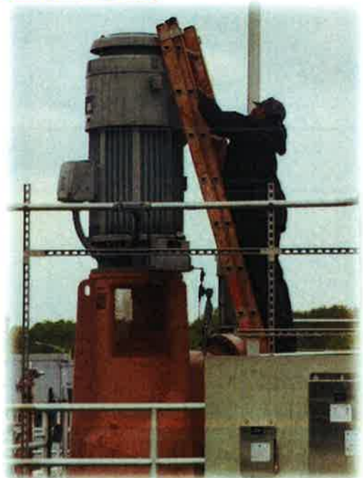
PREVENTIVE MAINTENANCE ON EFFLUENT PUMP
