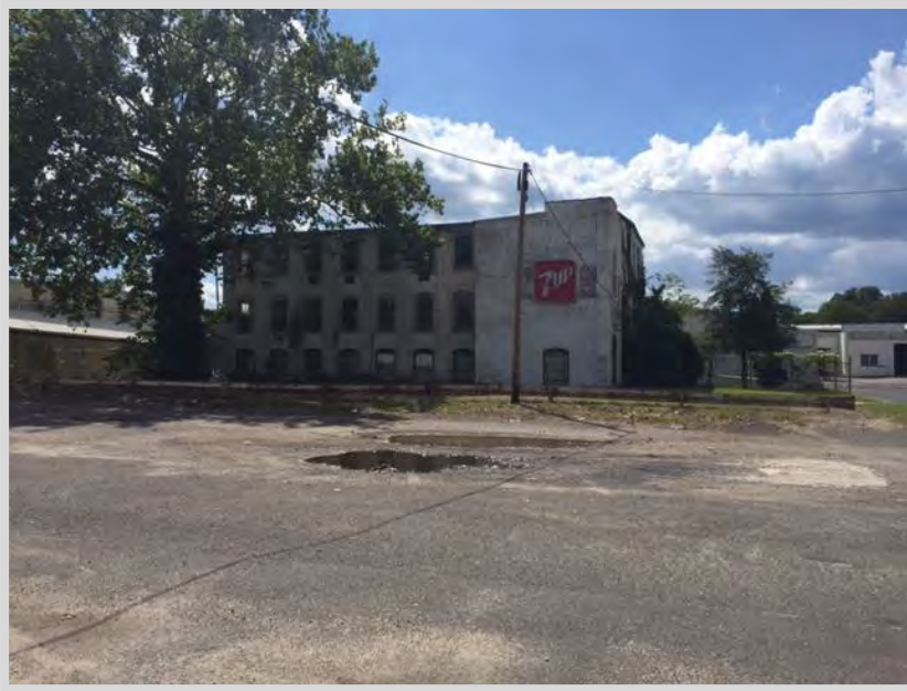
Vacant 7-Up building along the Cohansey River and Glass Street
