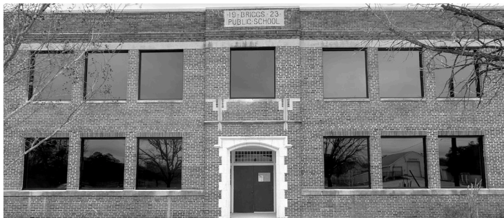
Work continues on the school building!
