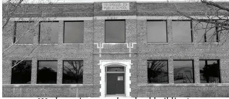
Work continues on the school building!
