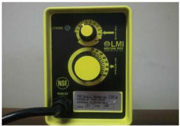
Prime and set pump for 1/2 gallon per day. Set pump at 30% speed and 30% stroke P121-353SI
