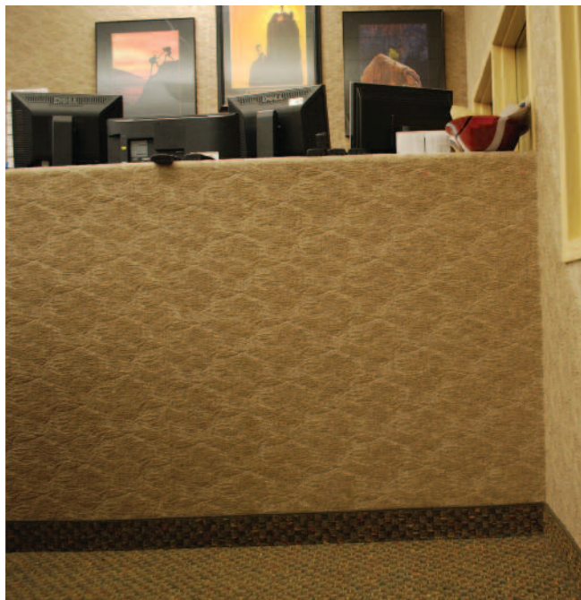
Hytex Industries Inc. uses 15 post-consumer PET bottles to produce each yard of its Eco-A.R.T. acoustical wallcovering. Doing so already has diverted an estimated 25 million bottles from the landfill. The end product also incorporates Fosshield, a patented antimicrobial technology from Foss Manufacturing Co. LLC. Courtesy Hytex Industries Inc.
