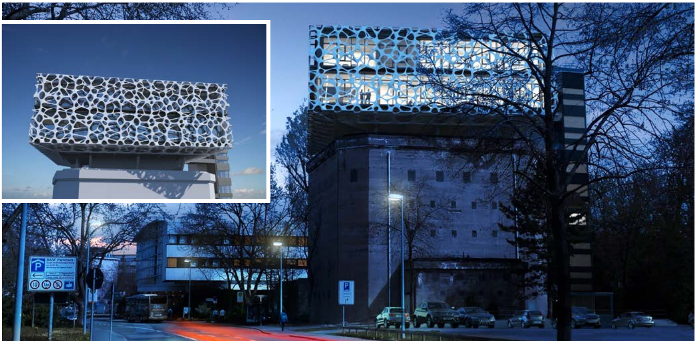
BASF's new Creation Center atop an old air-raid bunker on its campus in Ludwigshafen, Germany. The so-called "innovation factory" is designed to stimulate collaboration. Courtesy of BASF
