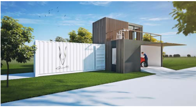
Gazelle Tech's modular microfactories ship in six 20'-long by 8'-wide shipping containers and cover about 1,075 square feet when assembled into an office and workshop area. (left) The microfactories are spacious enough to allow for assembly of the entire car. (right) Courtesy of Gazelle Tech
