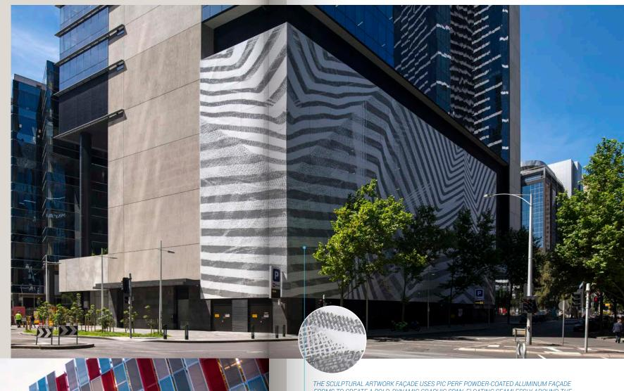
THE SCULPTURAL ARTWORK FAÇADE USES PIC PERF POWDER-COATED ALUMINUM FAÇADE FORMS TO CREATE A BOLD, DYNAMIC GRAPHIC SPAN, FLOATING SEAMLESSLY AROUND THE PARKING GARAGE EXTERIOR. ACTIVATING THE SURROUNDING URBAN LANDSCAPE, IT PRODUCES ILLUSIONS OF DEPTH, LIGHT AND PERPETUAL MOVEMENT.
