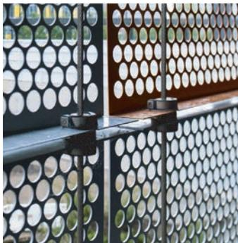
This project was to build a decorative facade and sunscreen that could also act as a pedestrian barrier for the new seven-level, 567-space parking building. In order to achieve greater installation efficiency and a more practical solution, we re-envisioned a design utilizing Atmosphere facade system after being approached by Thiess.
