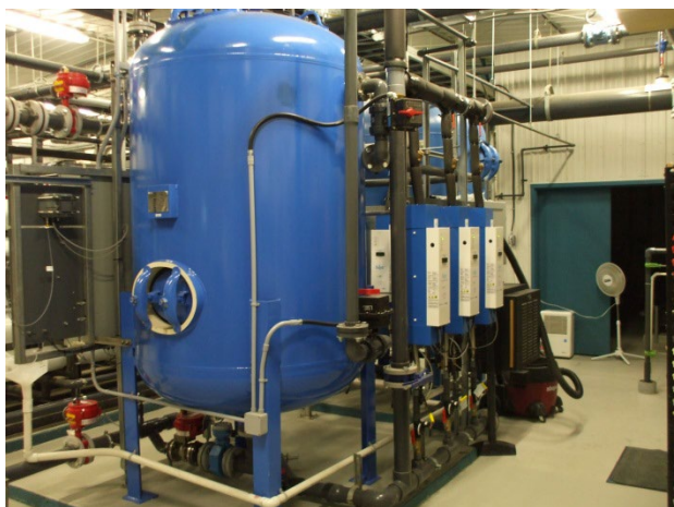
The New Sand Filter with UV
