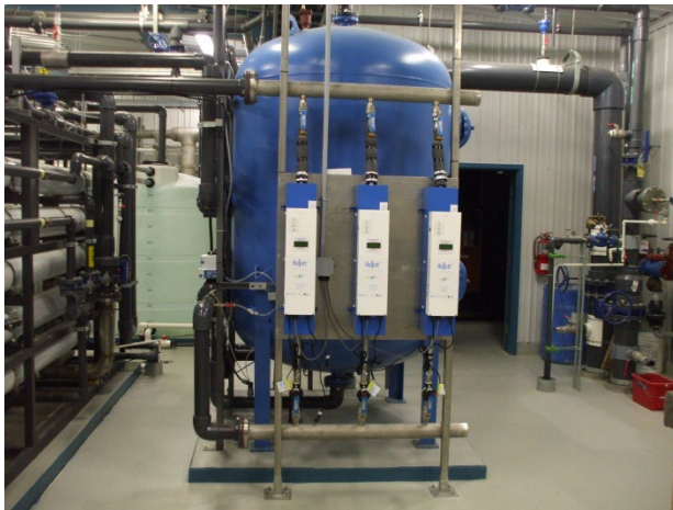
The Original Sand Filter with UV upgrade
