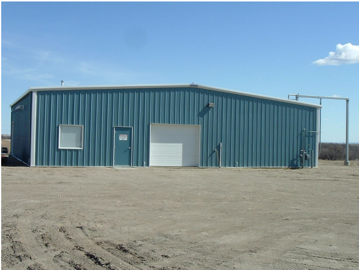
The Melita Water Treatment Plant
