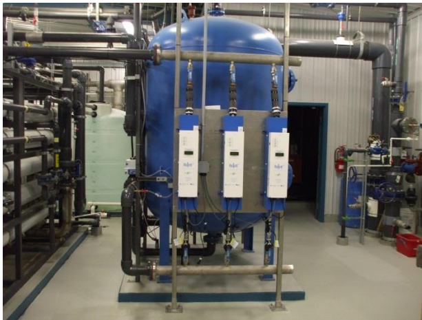
The Original Sand Filter with UV upgrade
