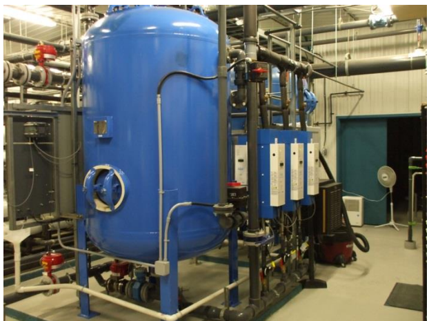
The New Sand Filter with UV
