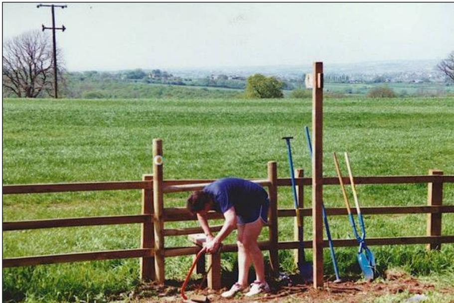
**A Trust member erects a stile and marker post on a Public Right of Way obstructed by a new fence.**
