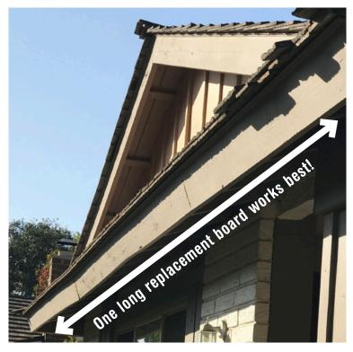
At right: Shown here is a 'bondo' type filler patch on a beam that has not stood the test of time—and now it is time for total wood replacement for this rotted beam, aesthetically and for proper structural support of overhead wood beams.
