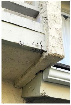
Above: Wood rot usually starts at the corners of wood planks where the water gets in, so be sure the new repair has the wood painted on all sides before installation.
