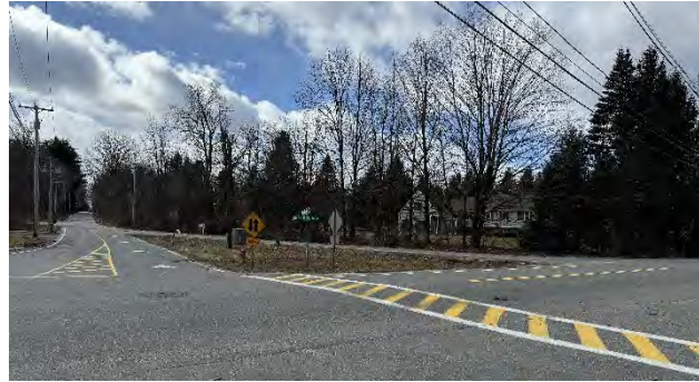
Figure 12-2. Geometric challenges, such as the Harvard Rd. flyway southbound from Seven Bridge Rd./Rte. 117, increase crash risks
