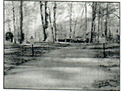
Existing Asphalt Driveway
