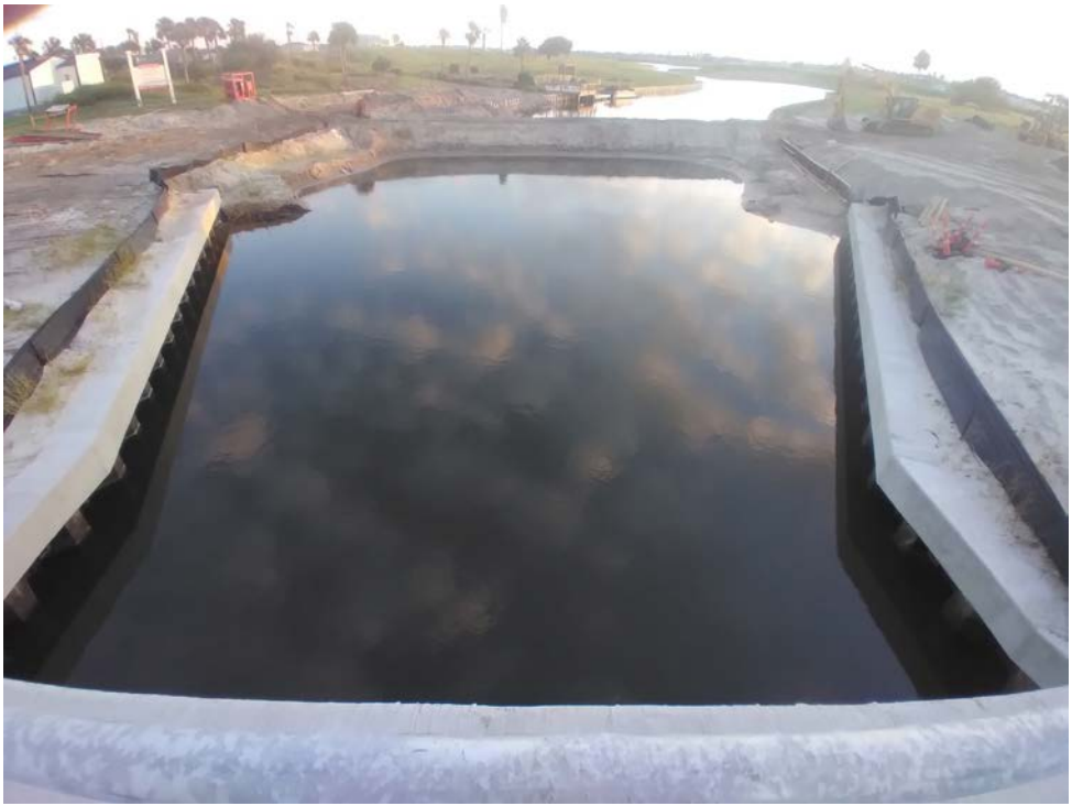
On the new Commodores Bridge looking south at the sand dam currently blocking the canal.
