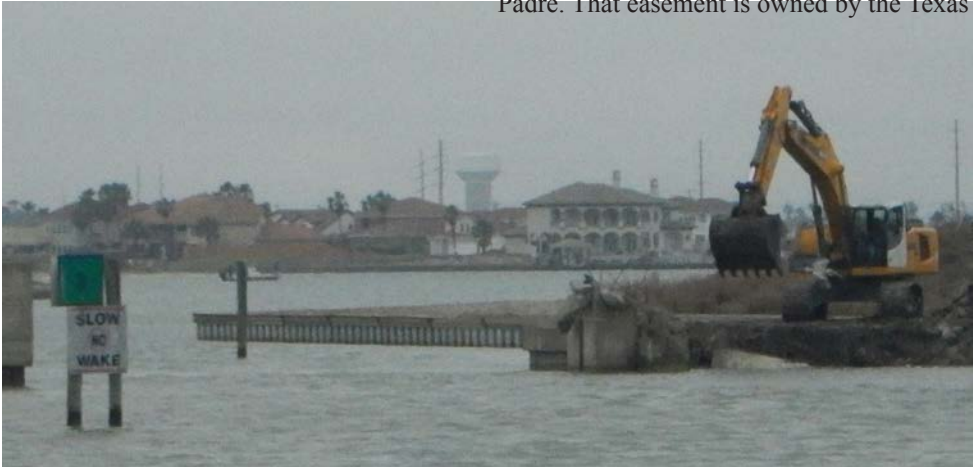
Demolition of the sea gate structure in 2020.
