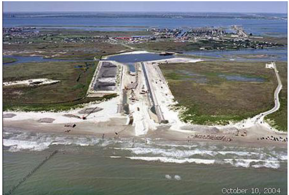
Packery channel under construction October 10, 2004.
