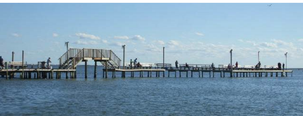
Red Dot Pier. Photo courtesy of visitcorpuschristi.com
