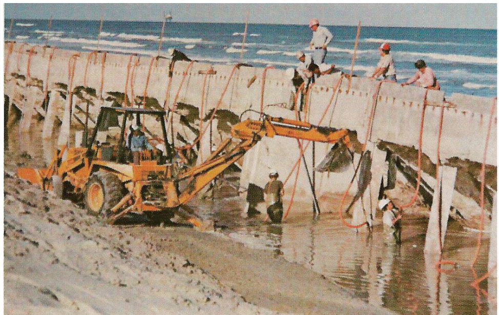
Seawall Repairs after Hurricane Allen damage
