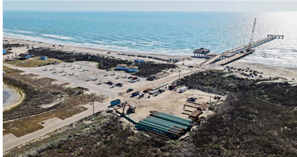
The Bob Hall Pier construction area
