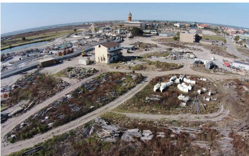
Ten years ago this week the Schlitterbahn waterpark was still a work site
