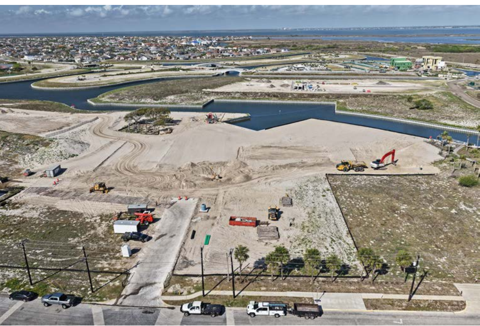
The Early Activation Center construction site
