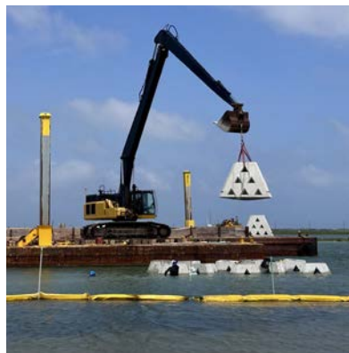
Reef structures for the living shoreline are dropped in place
