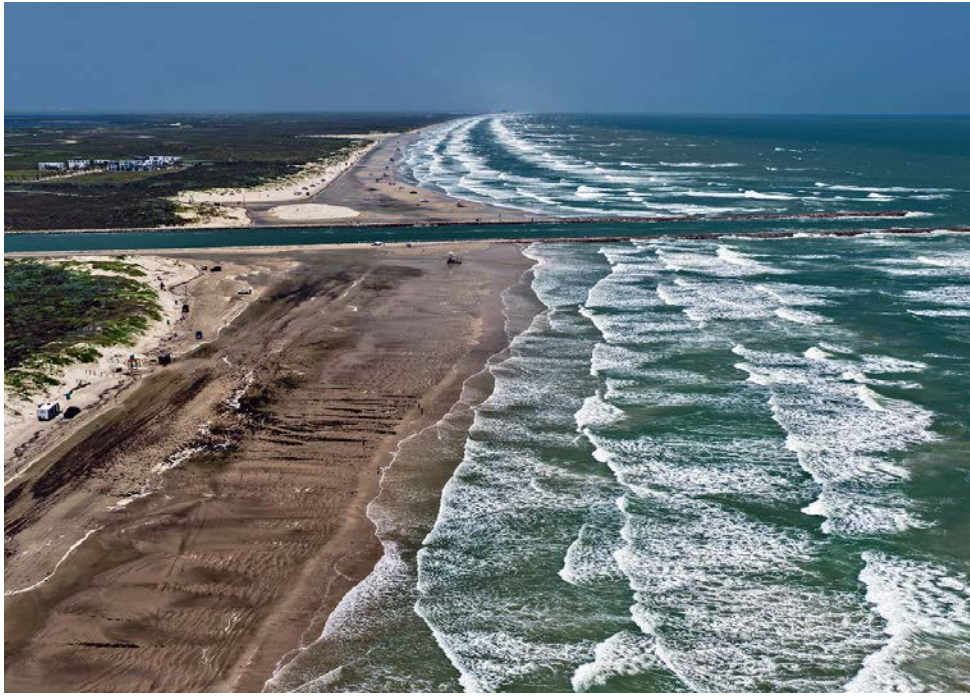
High winds and high tides have been around at Packery channel and the Michael J. Ellis Seawall. Aerials by Jacob Augs
