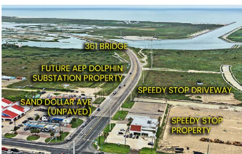
Park Road 22 at HWY 361 Intersection
