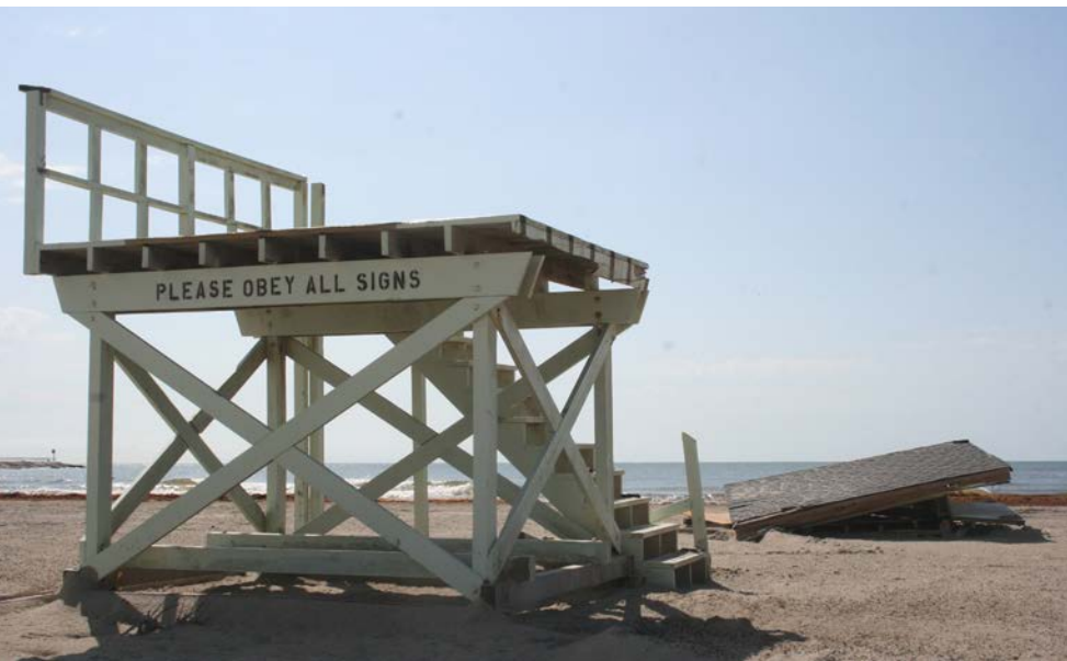
Hurricane Alex destroyed a few lifeguard stands
