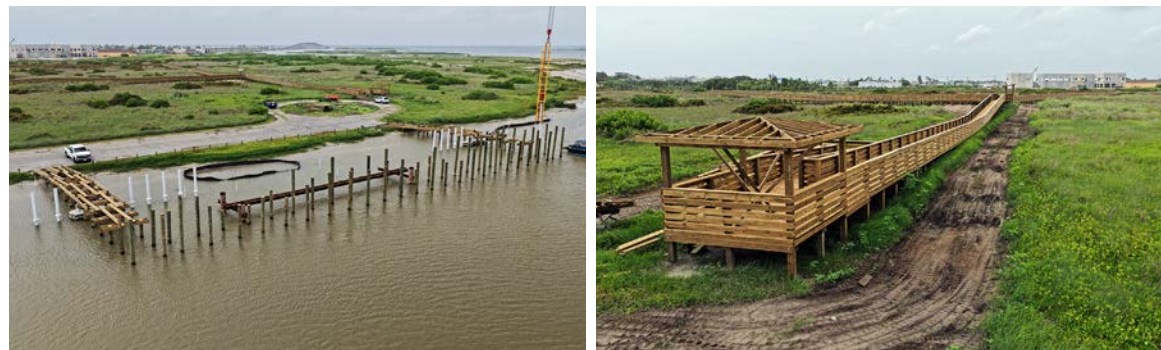
The Packery Channel Park fishing pier, boardwalk and living shoreline are well under construction. The nature park includes more than 1000 plants and trees, construction should be completed by the end of the year. More photos on page A2
