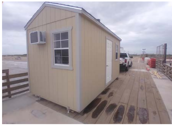
The new admission building is up at Bob Hall Pier but not yet in operation.
