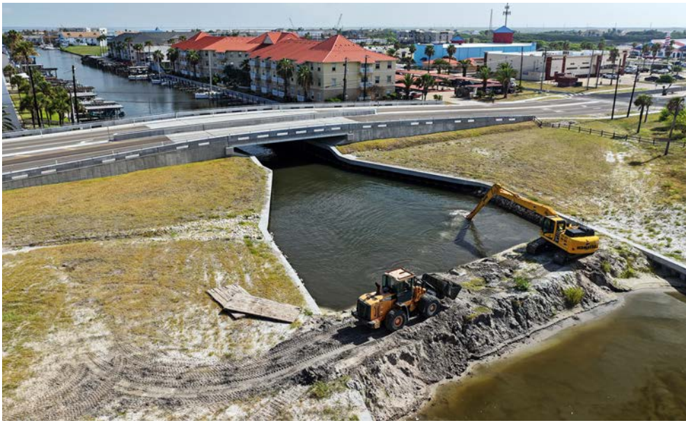
Crews working on the sand dam by Commodores Bridge
