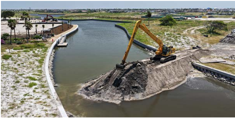
Work crews at the sand dam mid week
