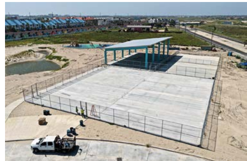
Commodores Park Construction
