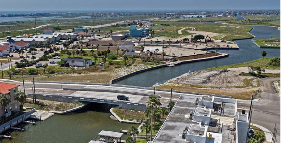
The Commodores bridge dam was removed recently
