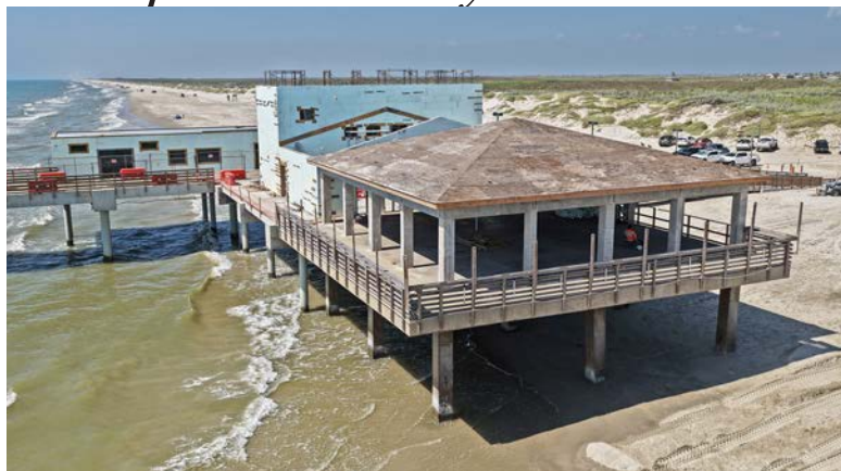
Work continues on the Bob Hall Pier restaurant
