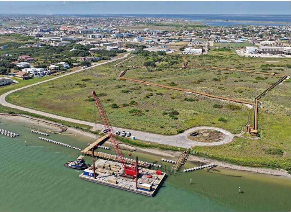
Work continues on the fishing peir and the walkways at Packery Channel Park. Work should be completed by the end of the year.
