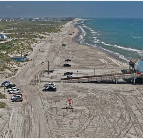
The current condition of the road in front of Bob Hall Pier
