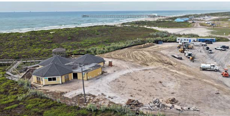
The old Briscoe King Pavilion and Bob Hall Pier
