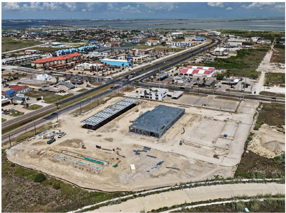
Work continues at the Speedy Stop on the Island. The access to Highway 361 is under construction on the right, and the car wash, gas pumps, and convenient store are all moving along.
