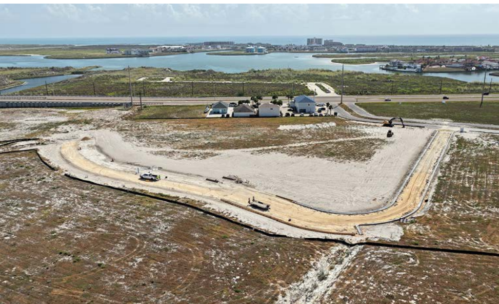
Work continues on the road to the Whitecap Marina off of Nemo court
