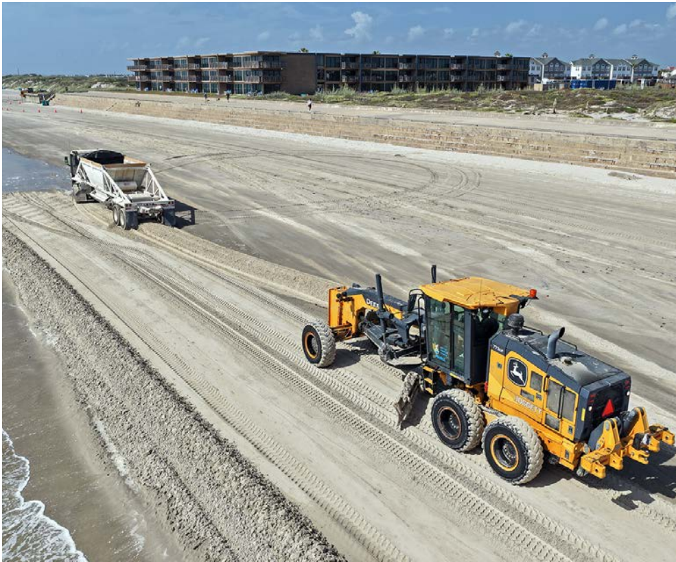
Beach renourishing continues in front of the Michael J. Ellis Seawall
